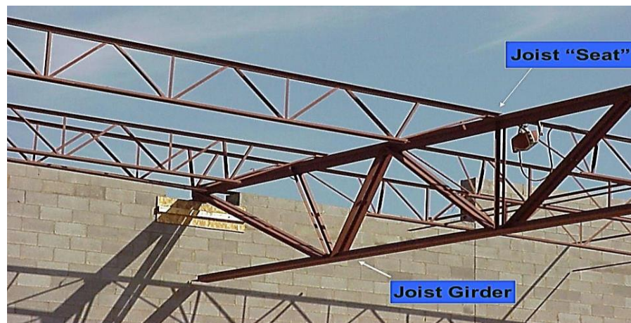
Figure 4-2-2 Joists
